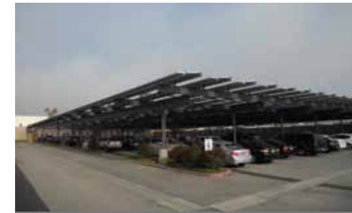
Solar panels deployed over surface parking lot at Downey Kaiser medical office building.
